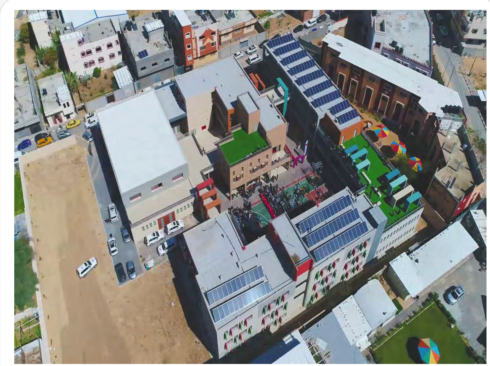
Jamal Abdel Naser secondary school, with 45 kWp installed PV system
