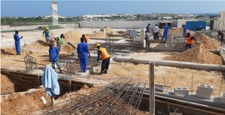
Construction work on the NIEC data centre and warehouse in progress and building is expected to be completed by the end of February 2020
